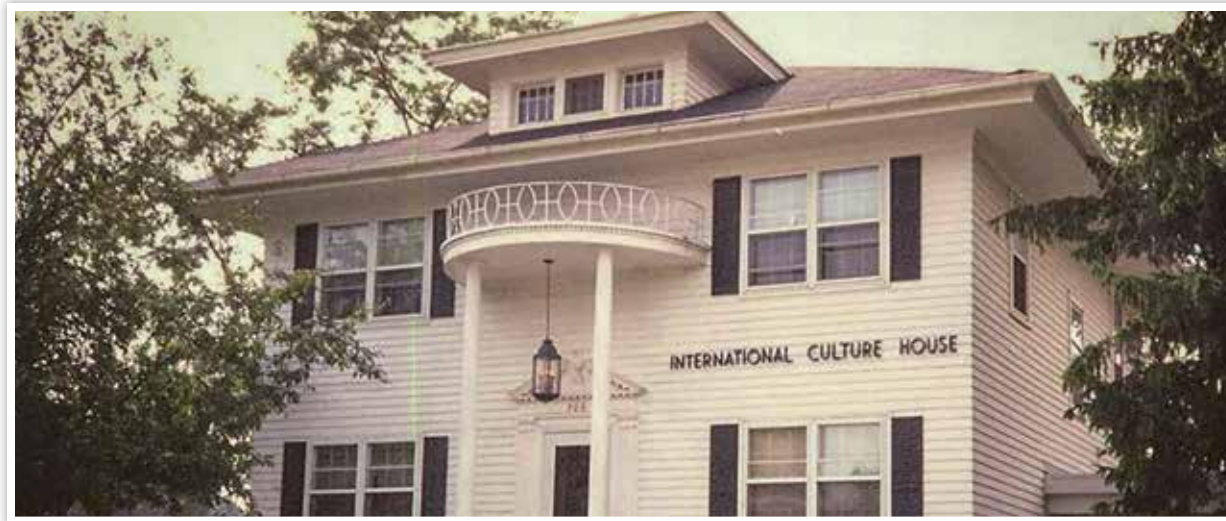
The house at 306 Third Street in the late 1970s.
